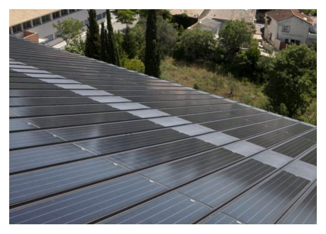
Figure 17 – Example of solar panels on zinc roof where the solar panels are installed between the seams of the zinc
